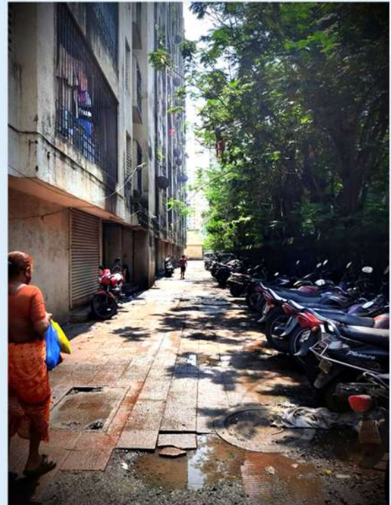
Dosti Complex, MMRDA Housing, Vartak Nagar-Thane West, Image courtesy-Esha Gupta
